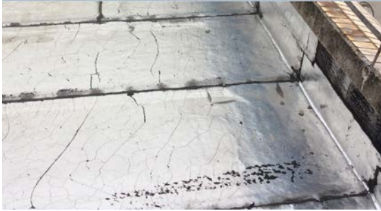
Figure 1: A sample of modified bitumen roof membrane with aluminum silicate coating.
